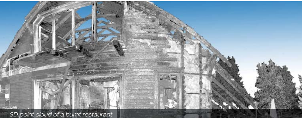
3D point cloud of a burnt restaurant
